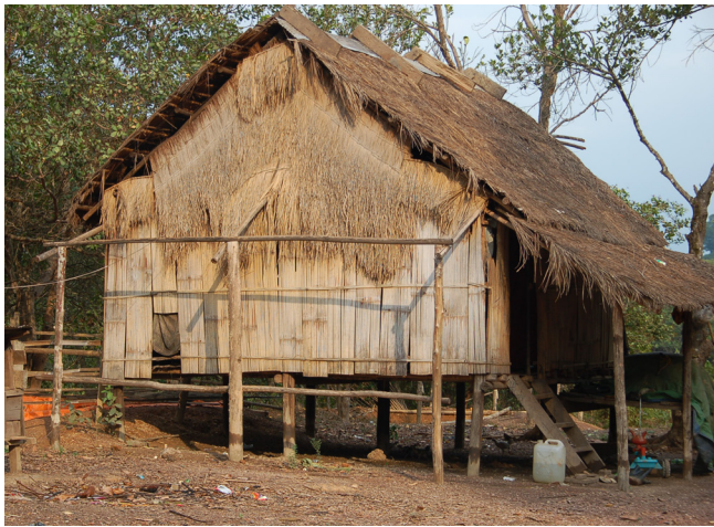
Typical dwelling of local communities in the Mondulkiri Province, made entirely of timber and non-timber products from the surrounding forest
