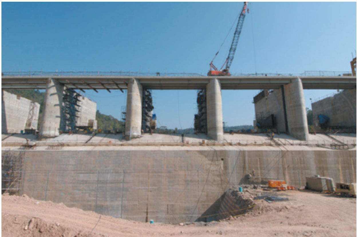
Sluice gates under construction at the Nam Theun 2 Dam. Photo: © Marcus Rhinelander
