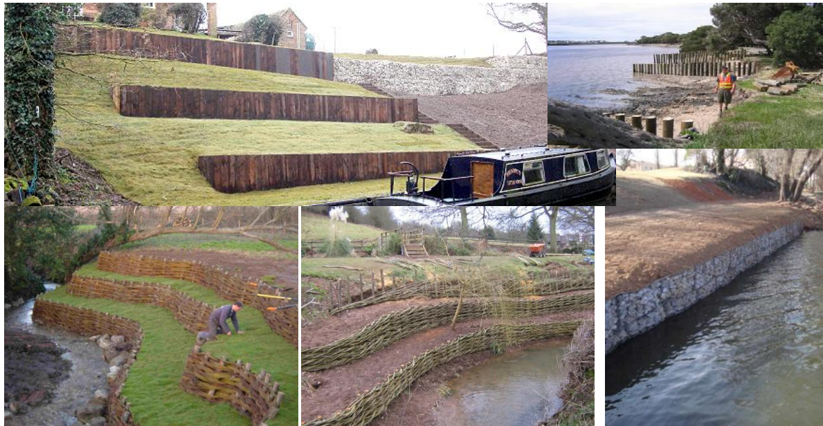
Figure 23: The canal banks - examples of stabilisation and vegetation bio-engineering techniques that could be applied. Top right - treatment at canal entry to Mekong River to reduce erosion and create landing areas
