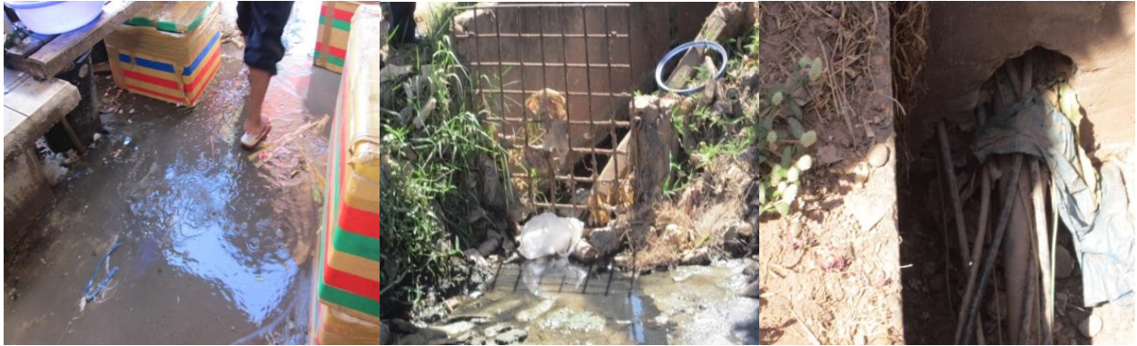
Figure 38: Savanxay Market area flooding (left), stagnant water (middle) and drainage being used to channel service lines (right), Kaysone Phomvihane
