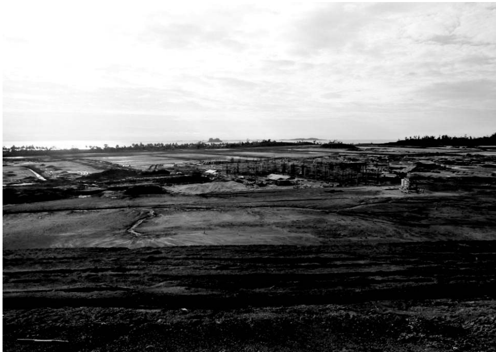
Onshore Gas Terminal being constructed near Kyauk Phyu.
