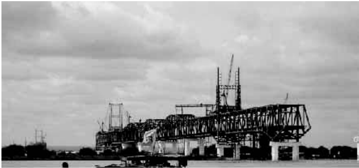
Ayeyawady Bridge (Pakokku) crossing the Ayeyawady River.
