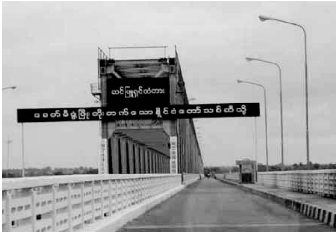
Sinbyushin Bridge crossing Chindwin River Source: MMRD Field Survey.
