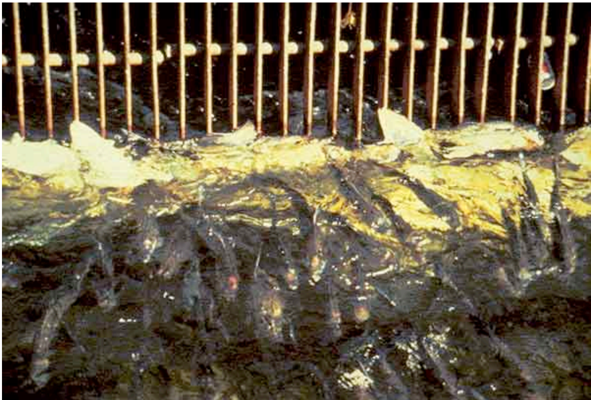
Figure 7-26. Impingement of Adult American shad on a powerhouse trash rack. Source: Larinier, 2001.
