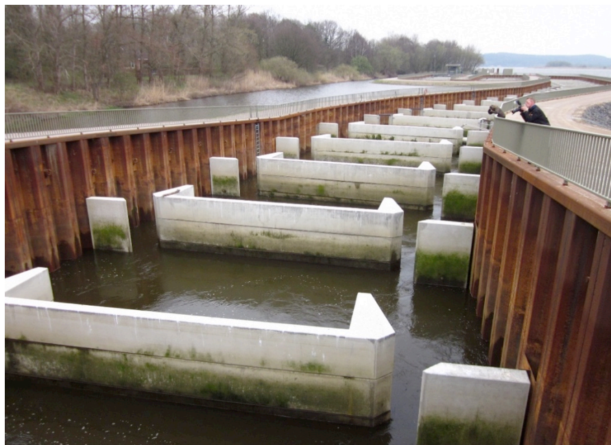
Figure 7-9. Example of a dual-slot vertical slot fishpass on the River Elbe in Germany. The proposed design for Sambor Alt_7 replicates the dual-slot three times (Figure 7-8) to ensure sufficient biomass of fish can pass.
