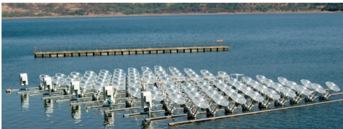
Figure 10-16. Sunenergy Liquid Solar Array, Tata Power hydro dam, India, with dual-axis tracking and concentrators.
