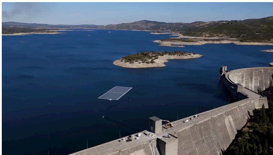
Figure 10-31. 218 kWp C&T, at Alto Rabagão dam, Portugal. Source: Moody's, 2017.
