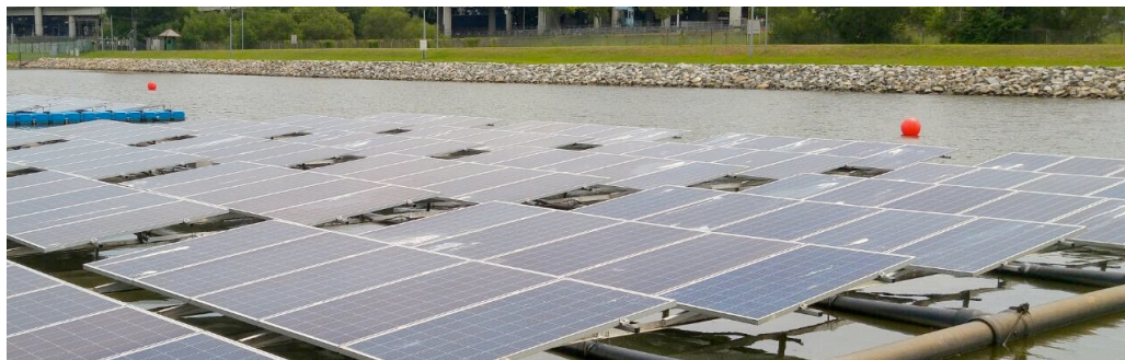
Figure 10-27. Bird droppings situation as observed at the Singapore floating PV Testbed.
