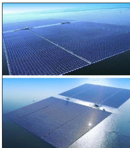
Figure 10-29. Basic building block of Sungrow floating PV arrays, with 2 units of 2.5MWac.
