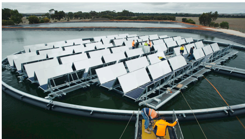
Figure 10-15: Infratech wastewater facility, Jamestown, Australia, with azimuth tracking (1-axis, vertical).
