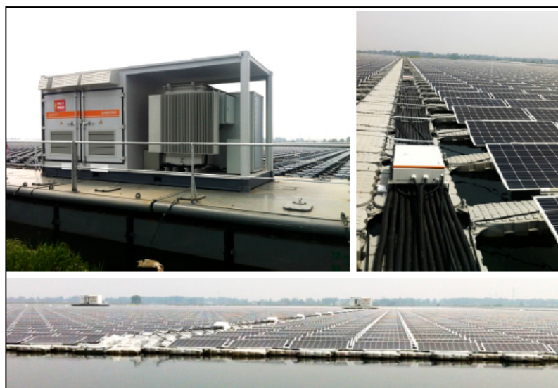
Figure 10-28. The standardized design for Sungrow floating PV system, with unit floating array block of 2.5MWac. The central inverter, switch gear and transformer are containerized and located in the middle of the floating array unit.
