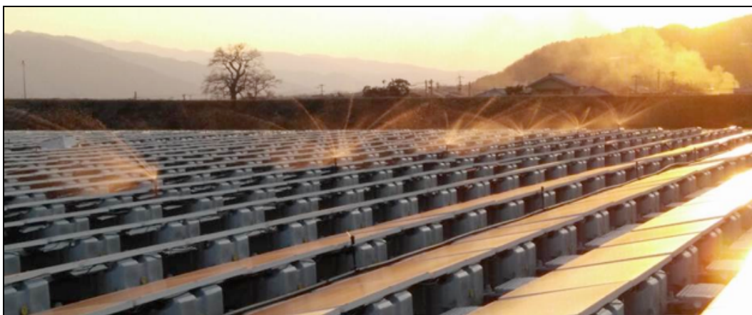
Figure 111-12: Floating PV system with active cooling, which may further enhance system performance and energy production (demonstration system built in Japan by Ciel et Terre).
