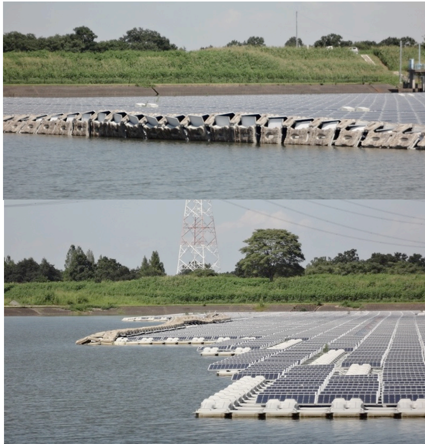
Figure 10-20. The damaged floating PV system, with its west "rim" turned over by strong winds and high waves. (source: Nikkei BP)
