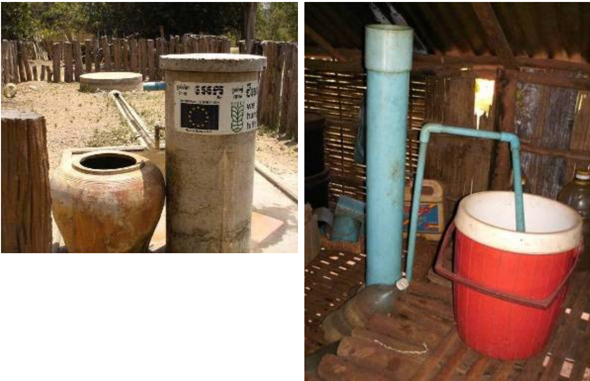
Figure 2.4.3. Left panel: Pumping house for drinking water in Kreung village in NE Cambodia constructed by Welt Hunger Hilfe and financially supported by the European Commission. Right panel: Sand-filter tube for drinking water purification in a household cottage in NE Cambodia; initiated by ICC. Photo: P. Stålnacke
