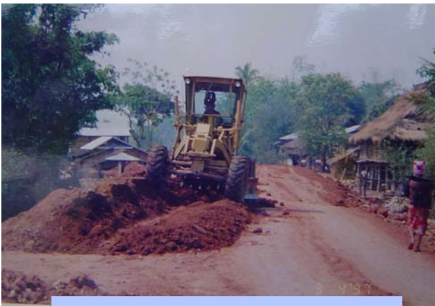
Construction of Road 17B in 1998
