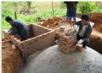
Photo 7: Biogas construction, Phoukout District
