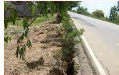
Figure 2-17: Embankment erosion (dragon hole) at NR1
