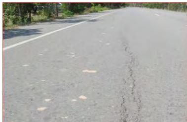
Figure 2-19: Longitudinal cracks at NR2
