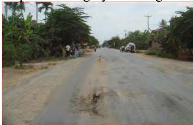
Figure 2-15: Loose foundation at NR21
