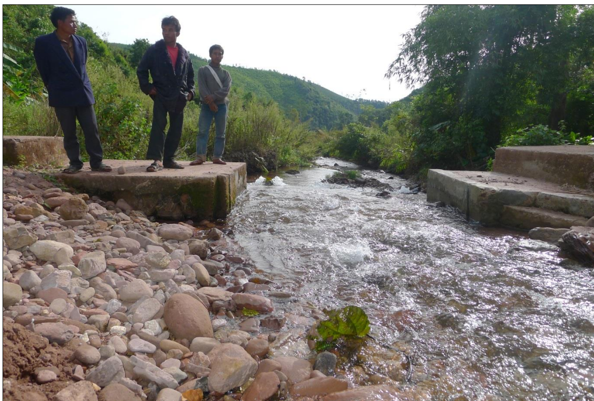
Satan villagers examine their repaired irrigation intake.
