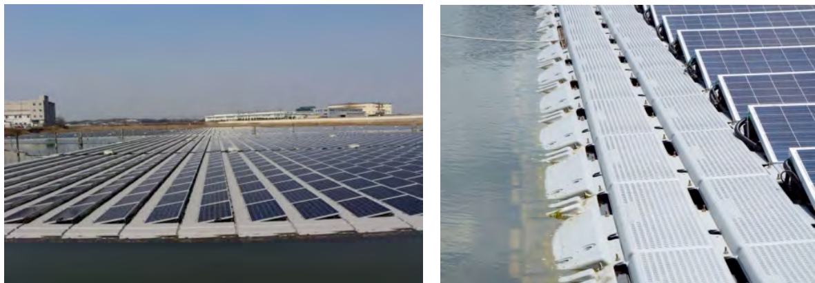
Figure 0-24. Ibiden's Floating Solar Mounting System.
