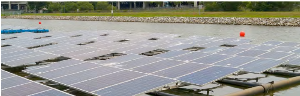
Figure 0-29. Bird droppings situation as observed at the Singapore floating PV Test bed.
