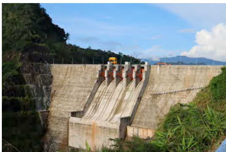
Figure 0-2. Xe Kaman 1: hydro power dam.
