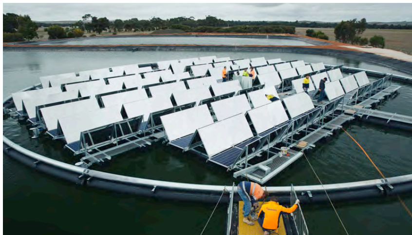
Figure 0-17. Infratech wastewater facility, Jamestown, Australia, with azimuth tracking (1-axis, vertical).
