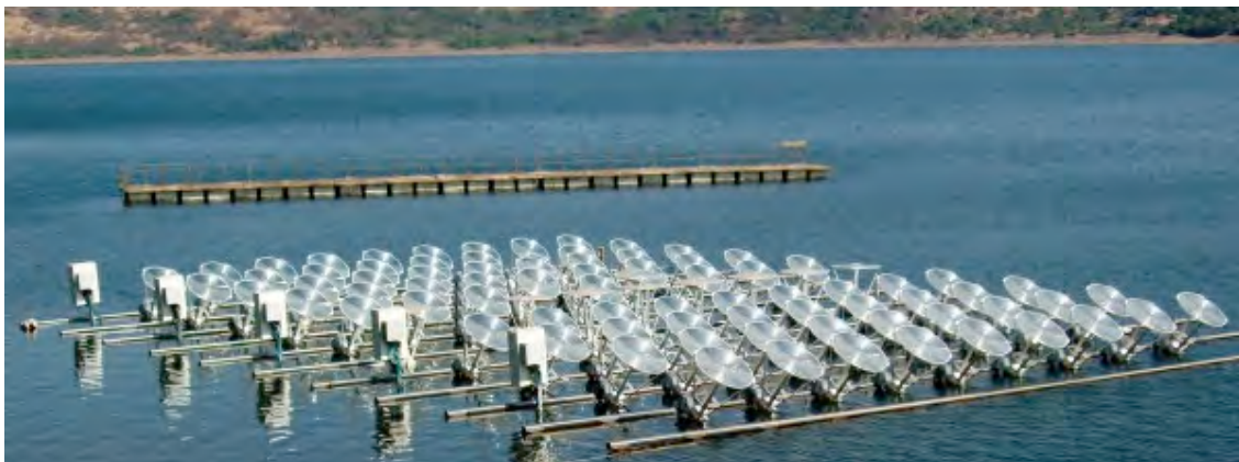
Figure 0-18. Sunenergy Liquid Solar Array, Tata Power hydro dam, India, with dual-axis tracking and concentrators.
