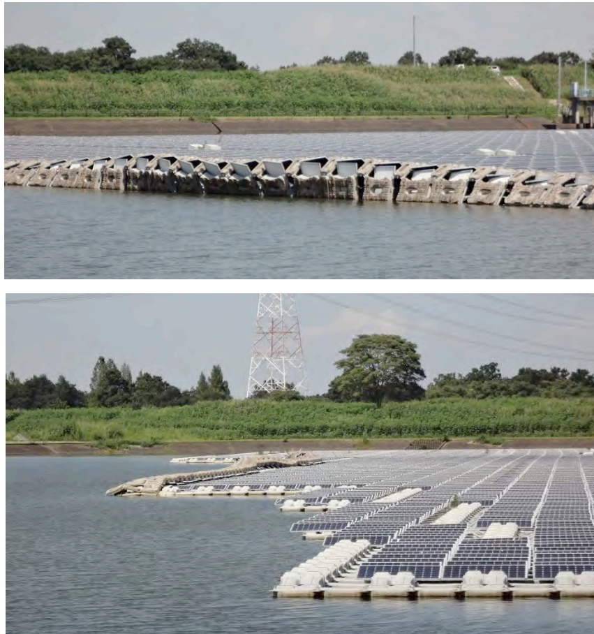
Figure 0-22. The damaged floating PV system, with its west "rim" turned over by strong winds and high waves (source: Nikkei BP).
