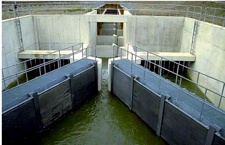
Figure 8-22. Fish screen at Iffezheim Dam, Rhine River. The screens direct fish into a vertical slot fish pass (centre), away from the turbine draft tubes. Photo: Marmulla (2001).
