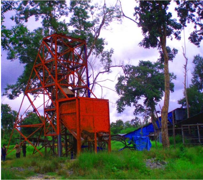
The Andong Bor Mine headframe
