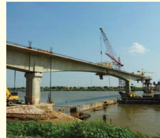
Construction of Prek Phnov Bridge
