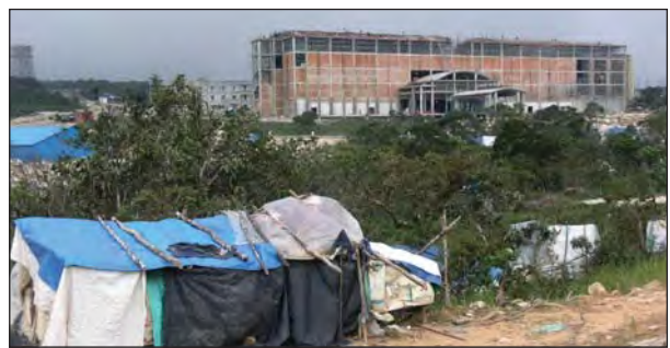
Fig. 4 The new casino under construction, on 18 August 2011 (© O. Kosterin).
