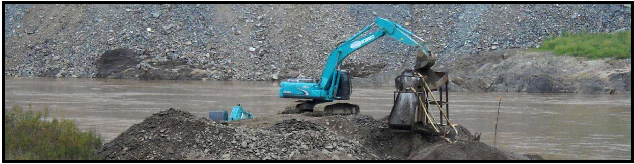
Construction activities at Xayaburi Dam Site, June 2012
