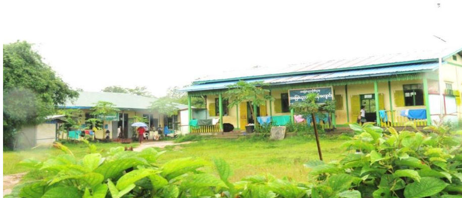
Figure-35: Primary school at Wat Kone Village
